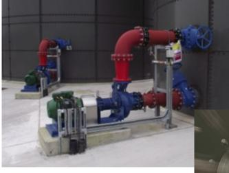
The Hidrostal screw centrifugal pump draws sludge from the source and returns it through a nozzle to provide optimum mixing energy and circulation of the tank contents.
